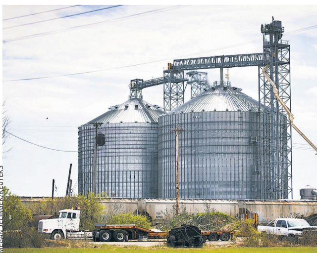
Storage tanks at a Cargill soybean processing facility in Ohio.
